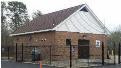
Water Dept. Filtration Building
