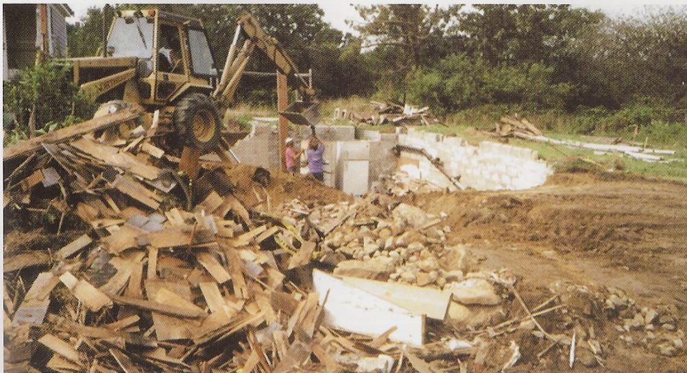
THE FOUNDATION WAS REMOVED, THE DEBRIS DISPOSED OF AND THE LAND SEEDED WITH NATIVE GRASSES TO START THE HABITAT RESTORATION PROCESS.
