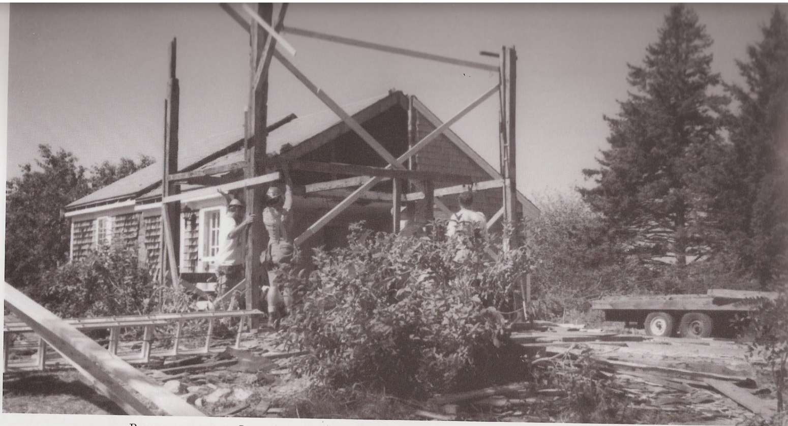
BOARD BY BOARD, CARL AHLSTRÖM AND LIZ PERRY ALONG WITH THEIR TEAM OF CARPENTERS DISMANTLE THE POST AND BEAM SEA CAPTAIN'S HOUSE BUILT IN THE 1840S.
