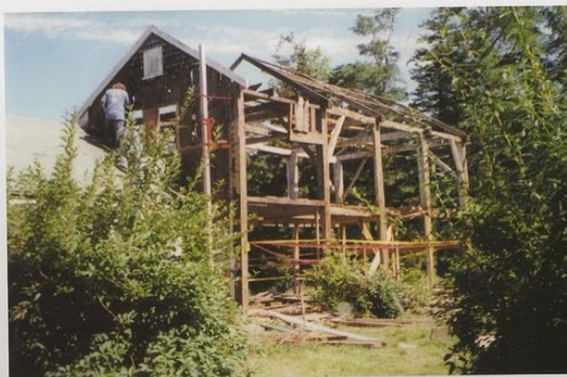
THE CAPTAIN WETHERBEE HOUSE IN BREWSTER (CASE STUDY #6) IS DISMANTLED BOARD BY BOARD IN ORDER TO CREATE A PUBLIC PARK. THE HISTORIC BUILDING WAS REASSEMBLED ELSEWHERE IN TOWN.
