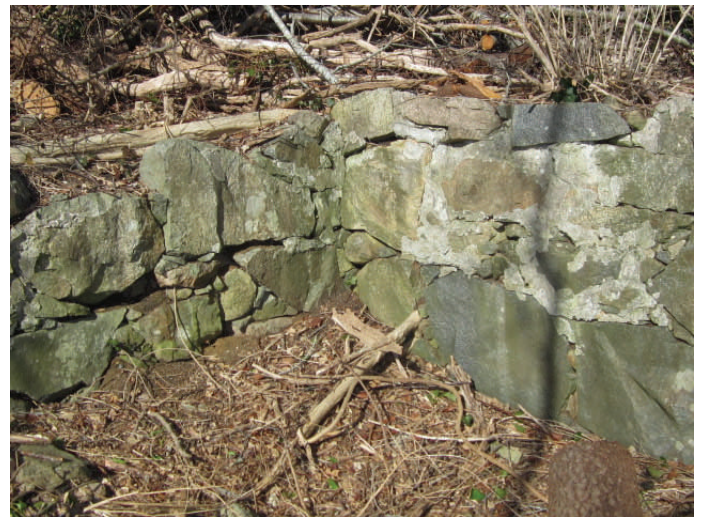
NE corner of rear wall
