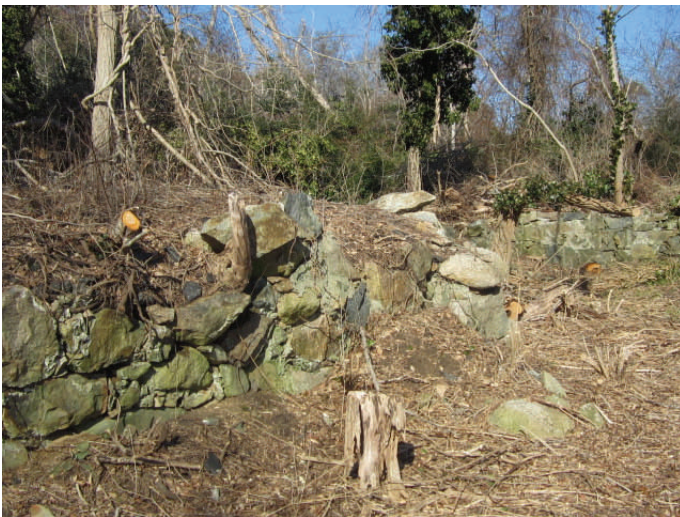
West wall in foreground
