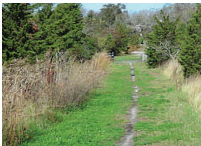
A walking path over Sea Street Dike connects Brewster & Dennis. The road was closed 30 years ago; the culvert was widened around 2007, allowing more tide upstream.
